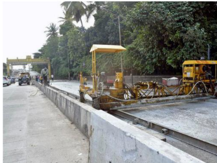
Mysuru road flyover down ramp closed for white-topping works in August 2021. K. MURALI KUMAR
