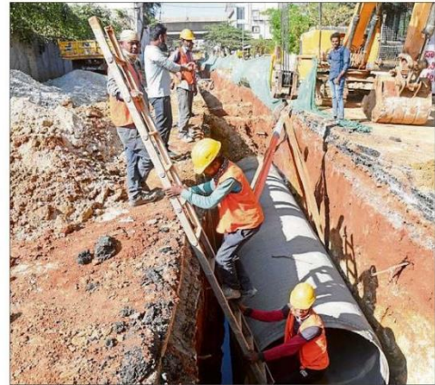
A file photograph of a pipe being laid to supply Cauvery water in Bengaluru.
