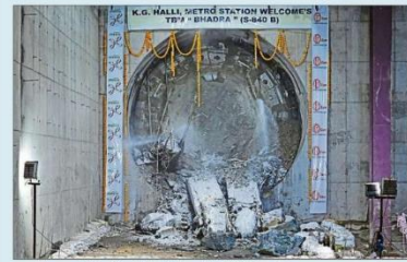
Tunnel Boring Machine (TBM) Bhadra emerges out of the Kadugondanahalli metro station.
