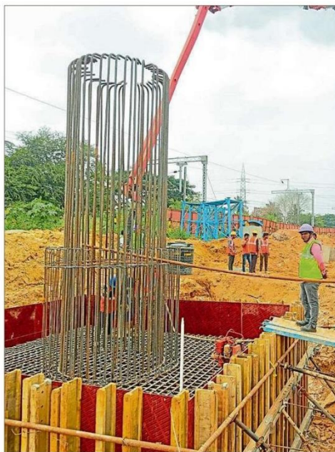
Concrete is being poured into a pile cap at Hebbal on the Bengaluru Suburban Railway Project's Corridor 2, the only line where groundwork has begun.. CREDIT: K-RIDE
