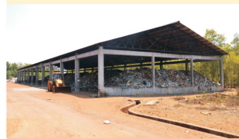
Alevoor Dumping Yard
