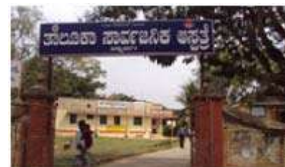
Taluka Hospital Byadagi
