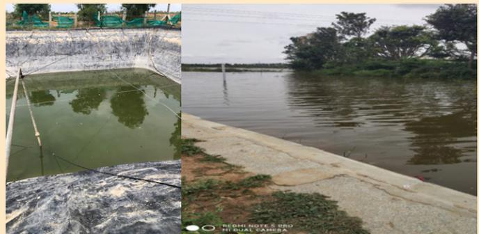
Farm pond lined with plastic film to store water. Kuratahalli minor irrigation tank filled with treated urban waste water from K C Valley project for recharging groundwater
